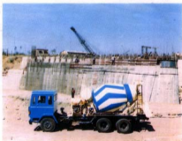
CONMIX truck mixer at Sardar Sarovar Namada Project
